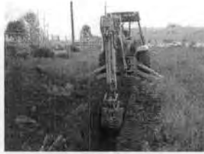
Figure 2. Trench 1, view to the east
