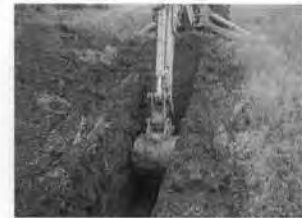
Figure 3. Trench 1, view to the east
