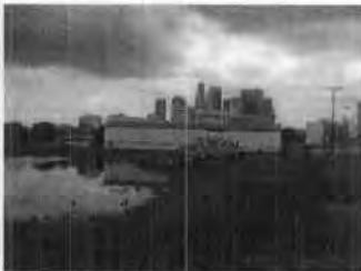
Figure 4. View to west
